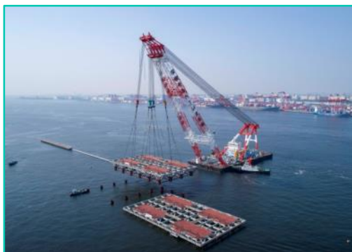
Construction zone #13 for new passenger boat wharf, quay, and parking area, etc.
