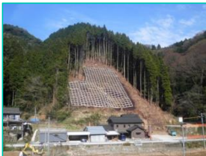
Construction at Tsuru Land Restoration Zone (Slope protection)
