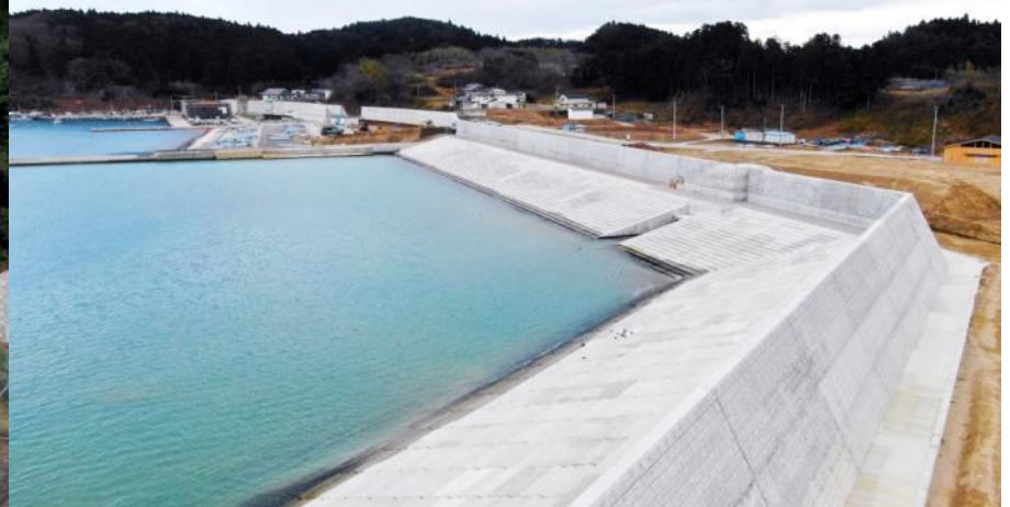
Mutsugaura Fishing Port seaside disaster recovery construction (Iwate Prefecture)
