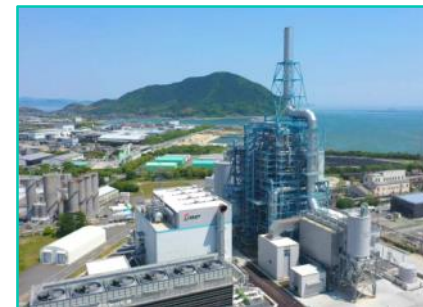
Hofu Biomass Power Plant construction (Heat retention, fire resistance)
