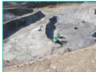
Koishwaragawa Dam construction (Blasting)
